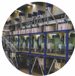
Advanced Processing & Milling
